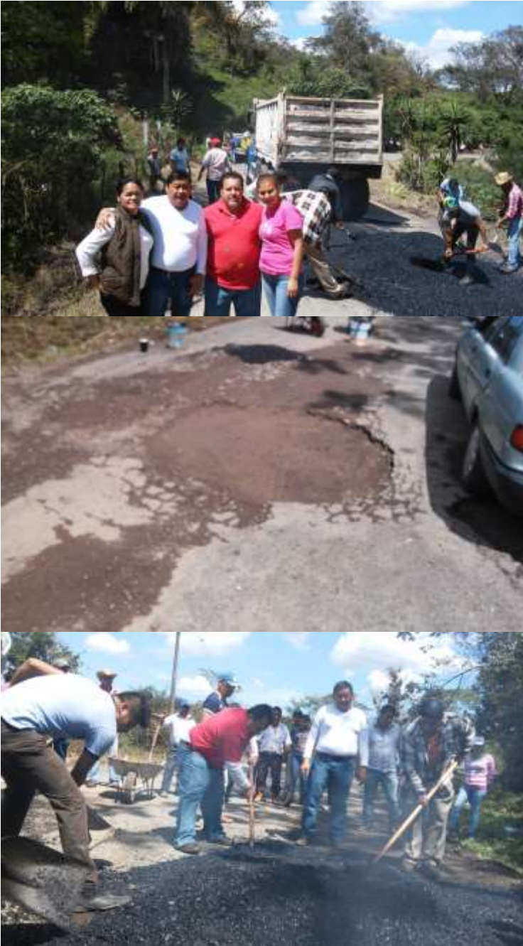
Bacheo carretera Huatusco-Elotepec.
